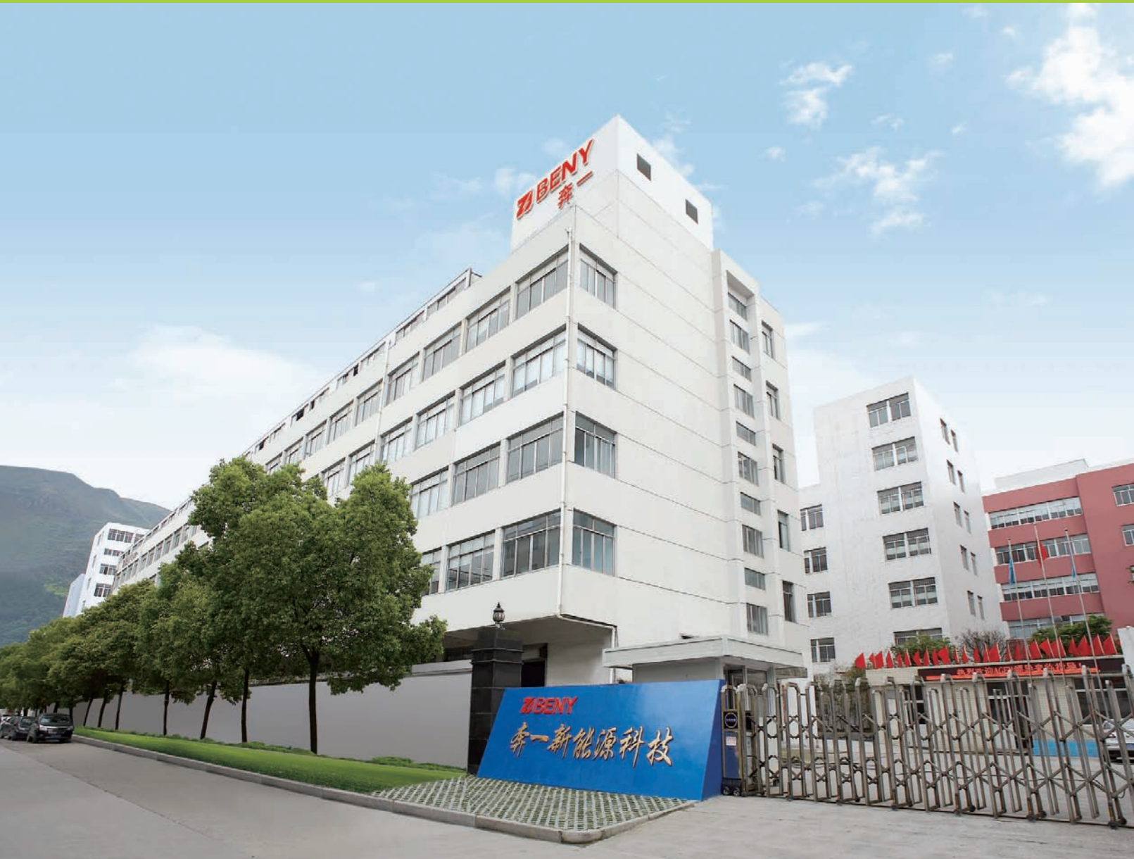
BENY Electrical Production Base in Wenzhou
